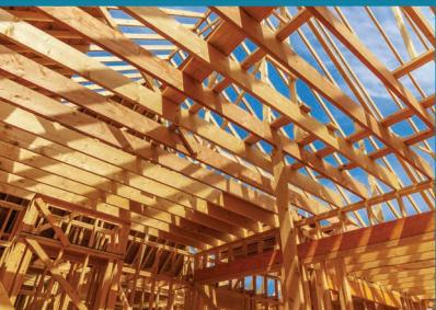
The concept of a wood frame construction that can function as an integrated unit and distribute load paths across its surface can be described as “monocoque,” or having a stressed skin design. This design concept is often used in aircraft engineering to create lightweight, super-
