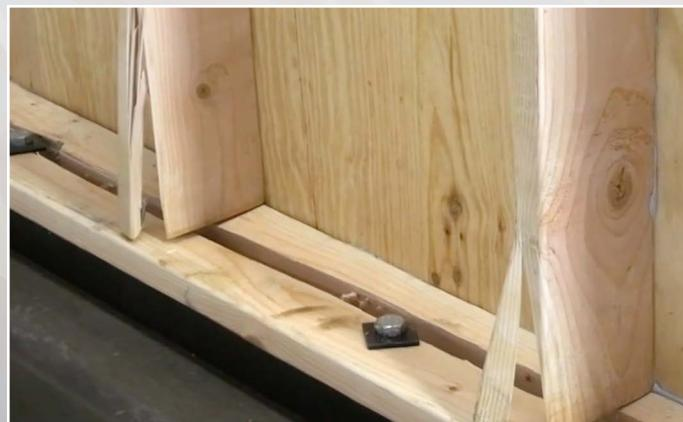
Climate Adhesive/Sealant NS applied to the interfaces between wood framing and sheathing can increase the structural integrity of a home by two to three hundred percent without weakening over time. This is accomplished without deviating from the Uniform Building Code at an estimate cost increase of only 1%.
